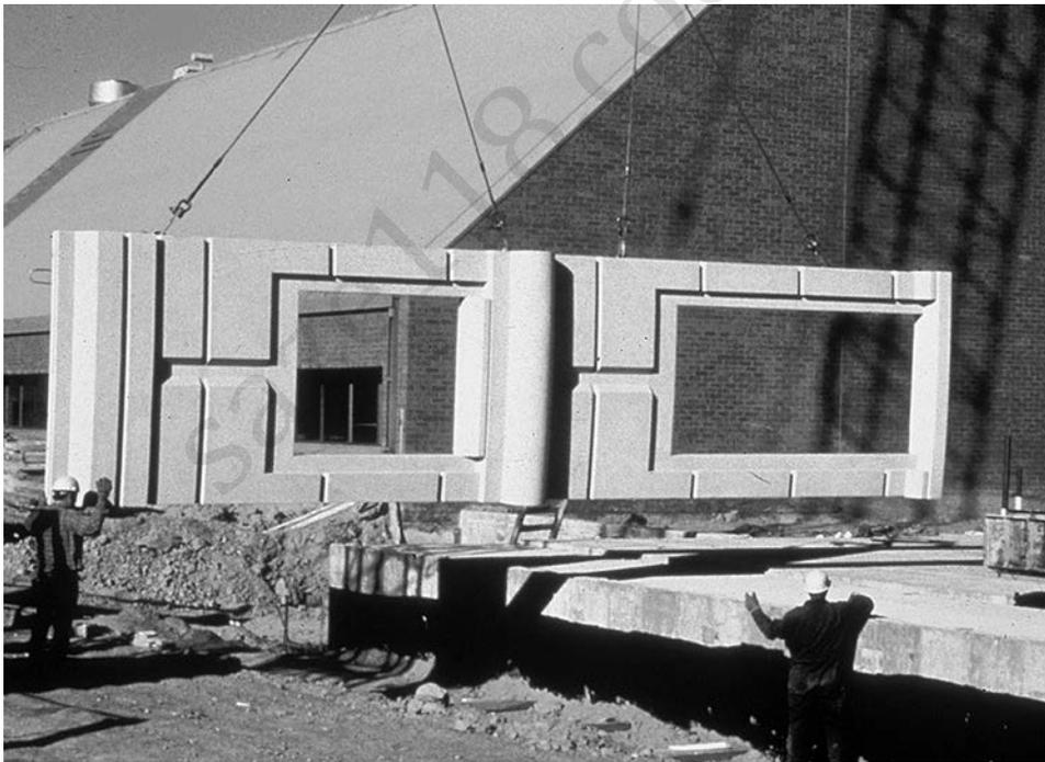
Fig. 6.2.1(b)—Panel stripped from mold.
