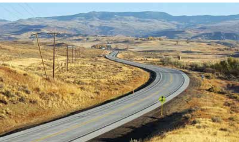
Colorado State Highway 13 was reconstructed using a 6 in. concrete overlay
