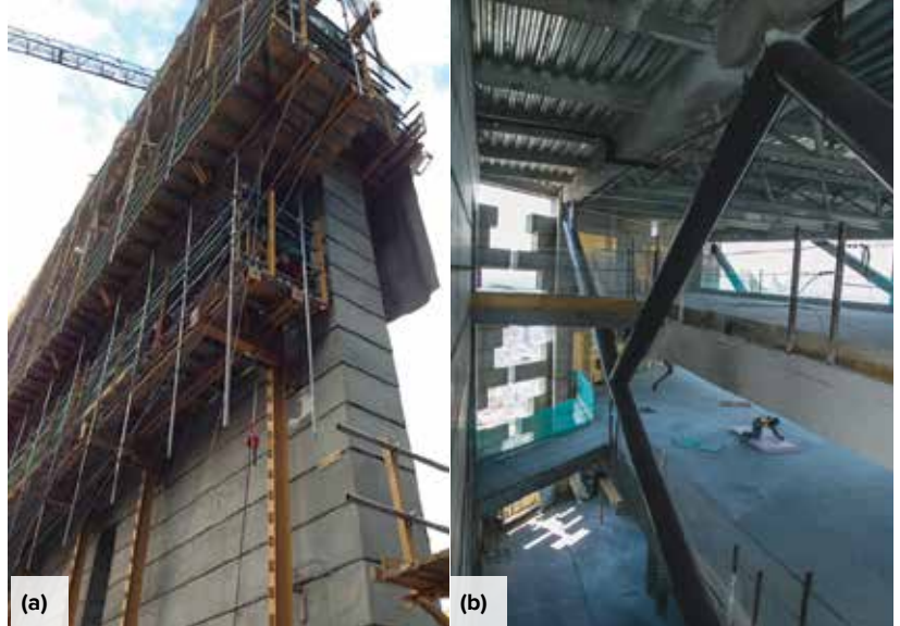
Fig. 3: Structural components of Torre Reforma: (a) shear wall formwork; and (b) atrium view of truss and perforated concrete shear wall
