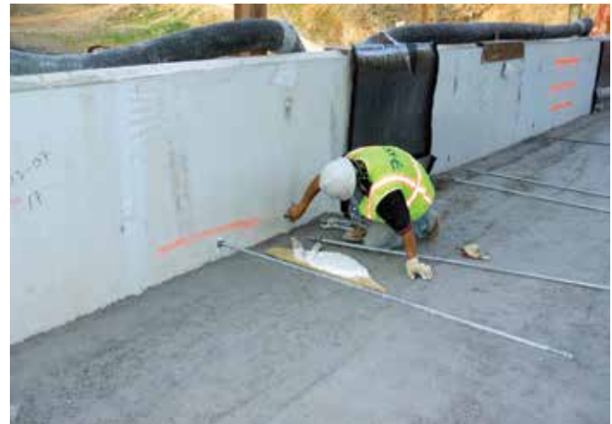
Fig. 7: Facing panel installation with anchors embedded between RCC lifts (© photo courtesy of Schnabel Engineering)
