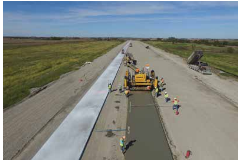
Sequenced paving lanes on the Northwest Missouri Regional Airport
