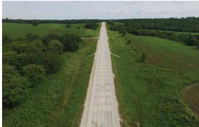
State Highway 52 was restored using patching and diamond grinding
