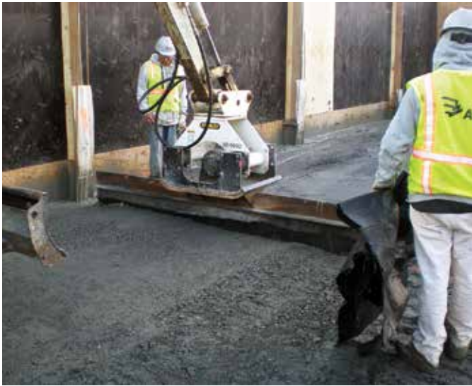
Fig. 11: Transverse joint construction by inserting and removing a plate in fresh RCC (© photo courtesy of Schnabel Engineering)
