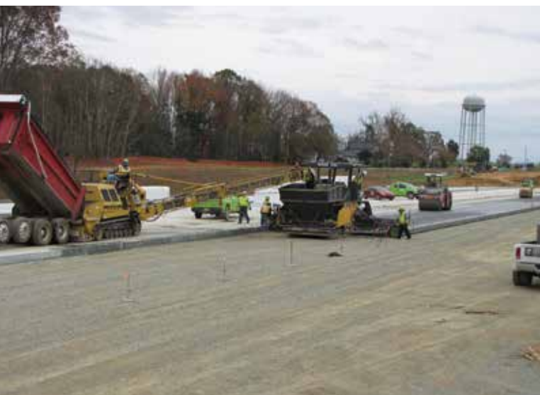
RCC construction at Walmart Distribution Center, Mebane, NC
