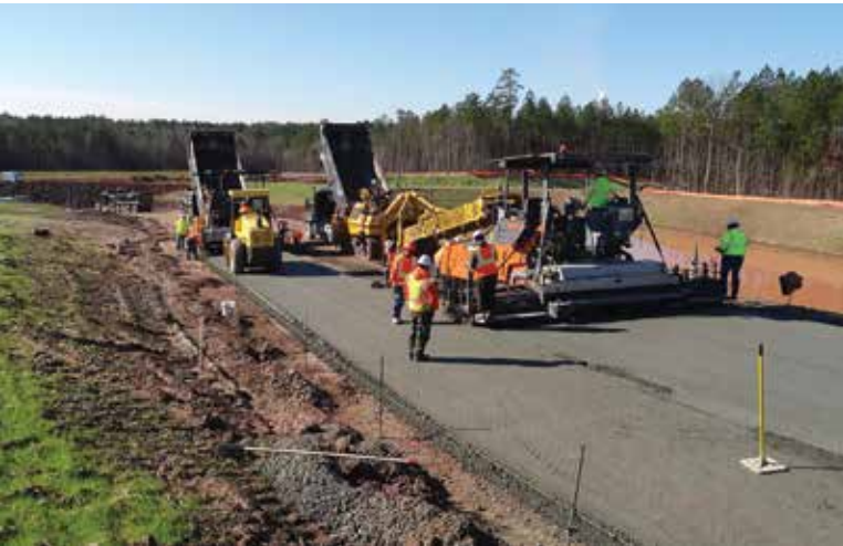
Placement of RCC pavement at the Brickhaven Ash Unloading Facility
