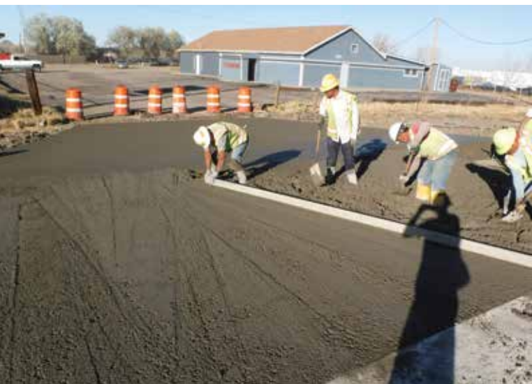
Colorado State Highway 119 was reconstructed using 9 in. dowelled concrete pavement
