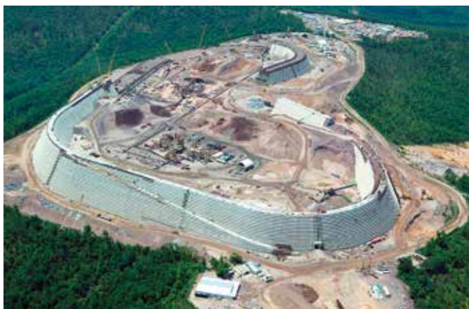
Fig. 2: Taum Sauk Dam, designed by Paul C. Rizzo Associates, Inc., is composed of several million yd 3 of RCC and with inner and outer facings of conventional concrete (photo courtesy of ASI Construction LLC)
