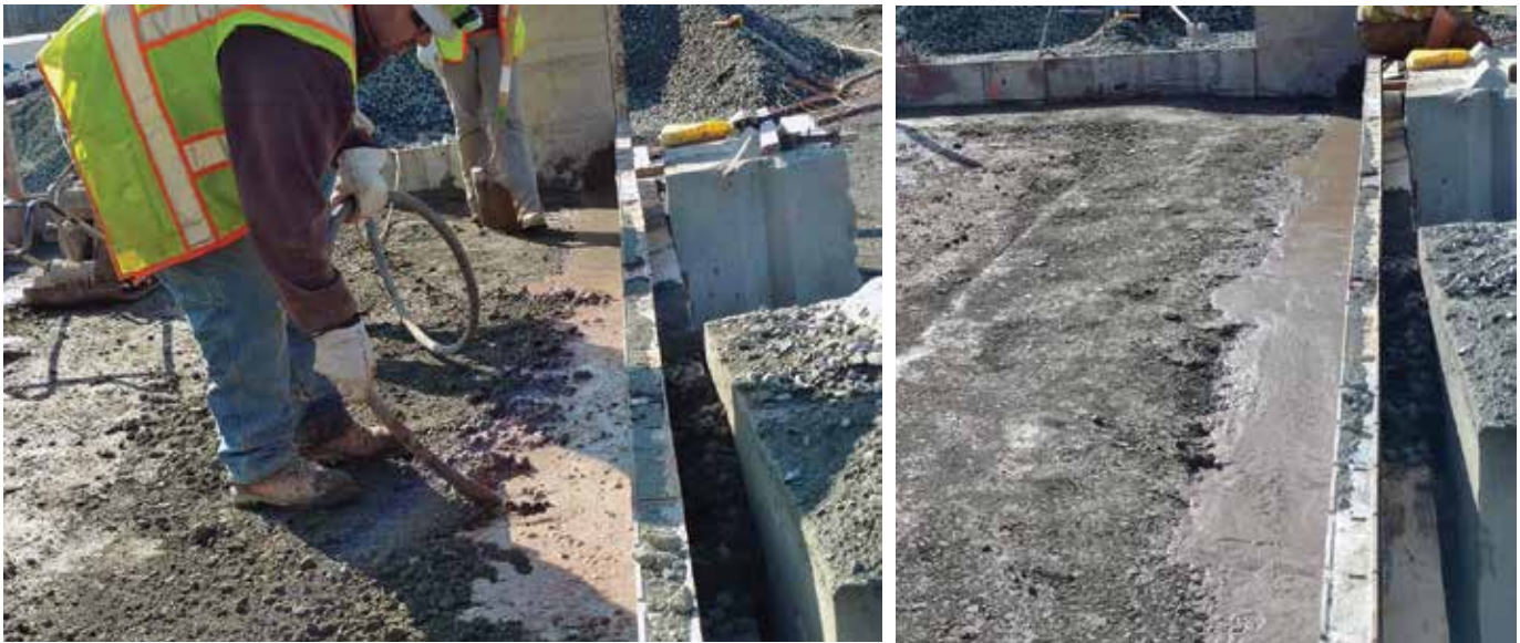
Fig. 6: A grout-enriched facing mixture is placed between previously placed RCC and formwork: (a) a mechanical vibrator is used to consolidate and combine the two mixtures; and (b) a completed test section (© photos courtesy of Schnabel Engineering)
