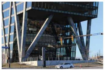
Fig. 6: The "tree columns" consist of three columns originating at a common node at the ground floor. Two branches inclined at 34 degrees from vertical support interior columns at level 6
