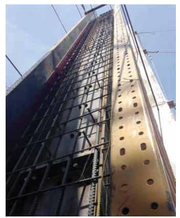
Ins act as both Fig. 7: Built-up structural steel core and deformed bars inside a tree column form (photo courtesy of DAVIS)
