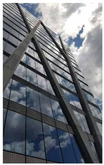
Fig. 5: The exposed concrete exoskeleton columns act as both braced frames and moment frames
