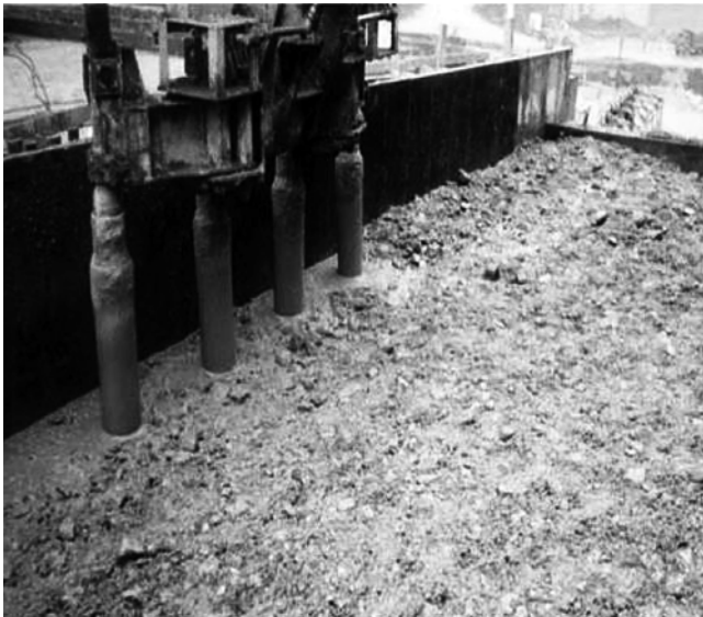
Fig. 6.15—GERCC: consolidating of GERCC by 6 in. (150 mm) gang-mounted immersion vibrators, Jianguya Dam, China (Forbes 2008).
