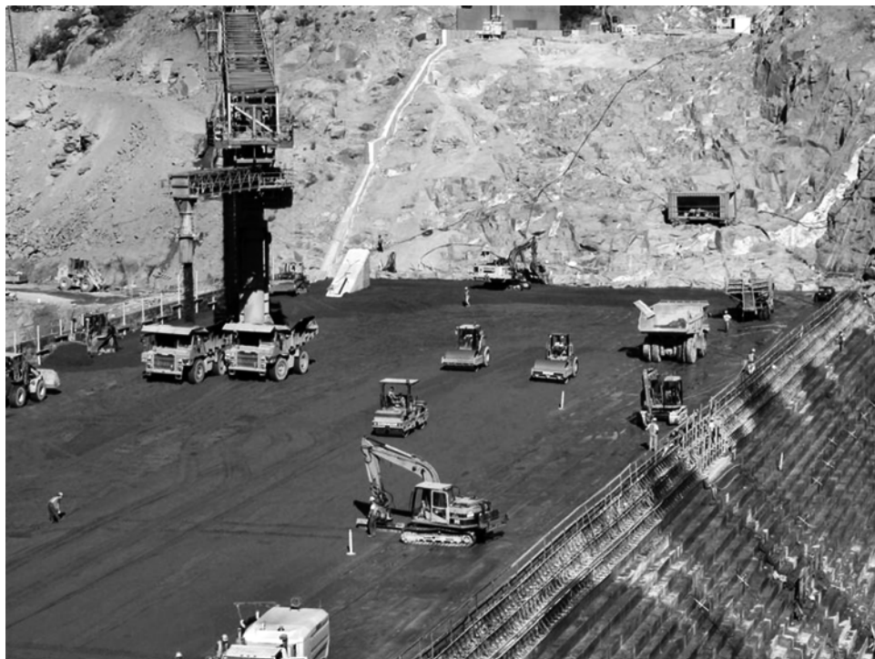
Fig. 6.3—Overview of RCC placement operations using conveyors transporting RCC from the batching/mixing plant to the dam body and transferred to end dump trucks, Olivenhain Dam, CA. (Photo courtesy of San Diego County Water Authority, 2002.)
