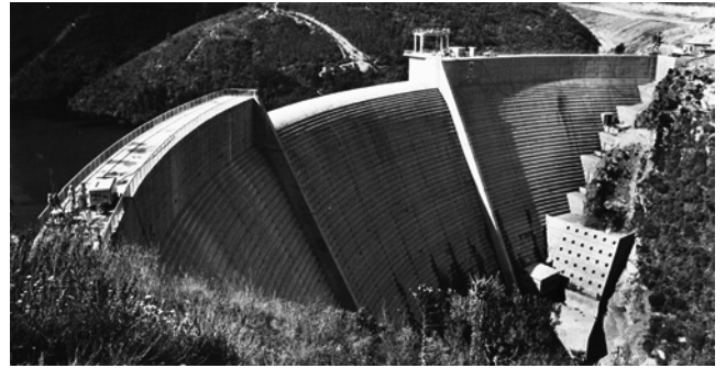
Fig. 1.9—Wolwedans Dam, South Africa (Hollingworth et al. 1988).
