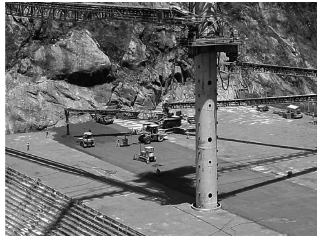
Fig. 1.7—Continuous all-conveyor placing, Miel Dam, Colombia. (Photo courtesy of INGETEC S.A., 2002).
