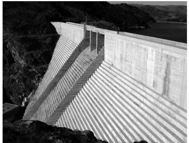
Fig. 6.12—Conventional cast-in-place concrete stepped facing, Toker Dam, Eritrea, Africa. (Photo courtesy of MWH Global, 2003.)
