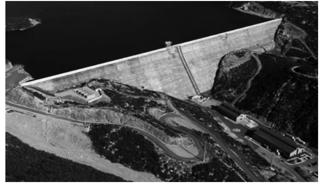
Fig. 1.6—Olivenhain Dam, CA. (Photo courtesy of San Diego County Water Authority, 2002.)
