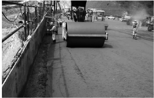
Fig. 6.16—Vibratory roller compaction at GERCC interface, Kinta Dam, Malaysia (Forbes 2008).
