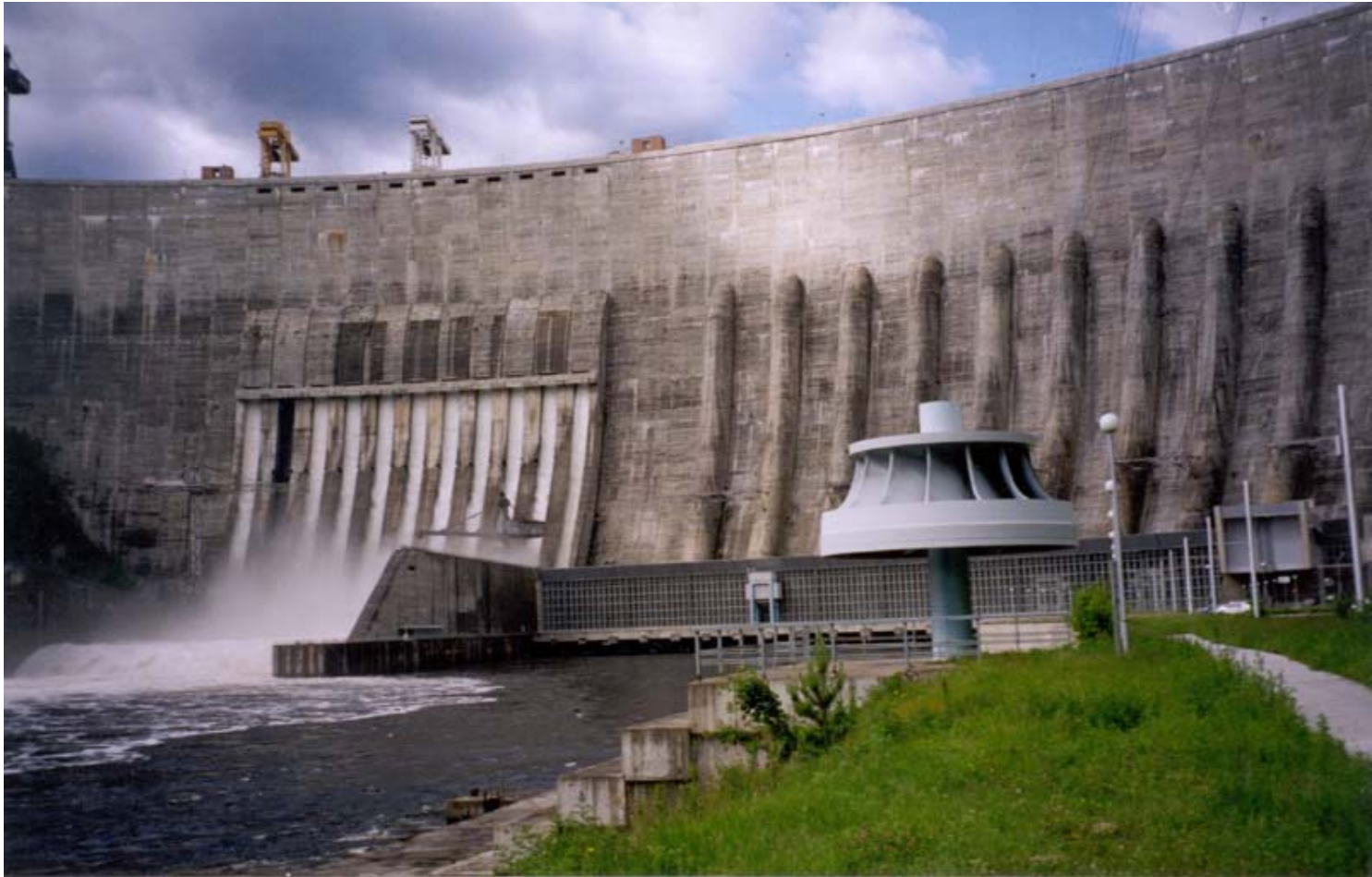
Fig.13. Concrete dam at Sayano-Shushenskaya hydroelectric plant (1982)
