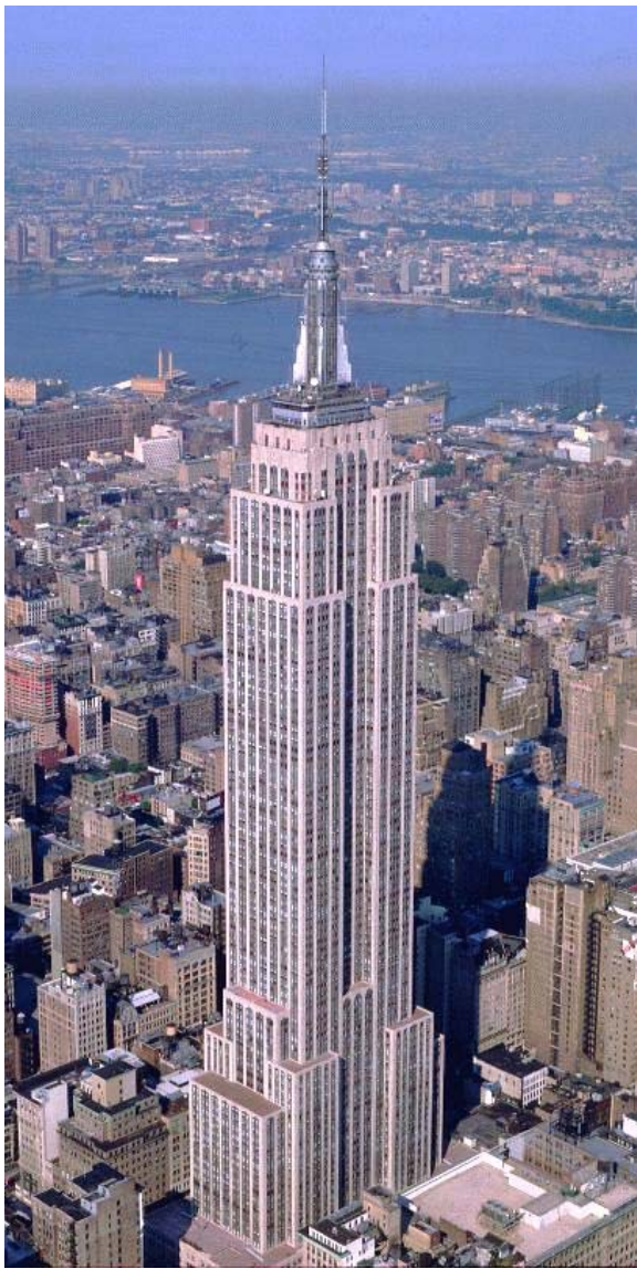
Fig.10. Empire State Building, New-York, USA (1931) 381 m high
