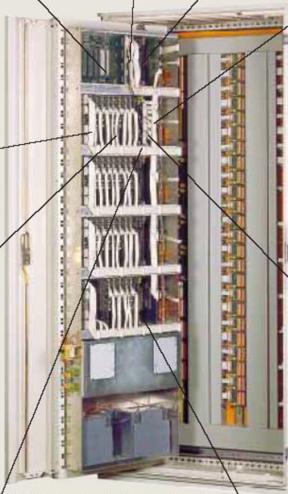
Fire detection and extinguishing control panel for 384 groups
