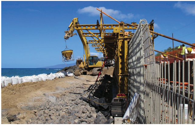
Fig. 3.2f—Construction of seawall with GFRP bars.
