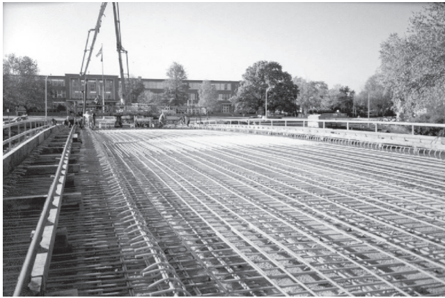
Fig. 3.2a—FRP-reinforced deck constructed in Lima, OH (Pierce Street Bridge), in 1999.
