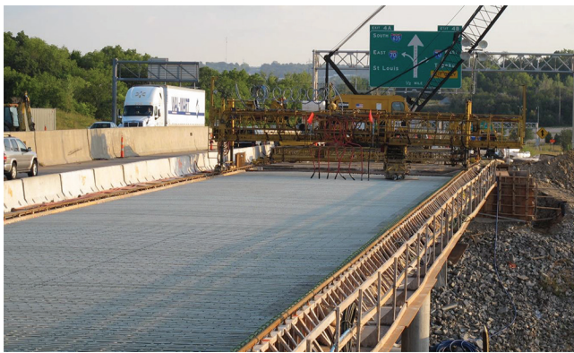
Fig. 3.2g—I-635 Bridge over State Ave. (Kansas City, KS).
