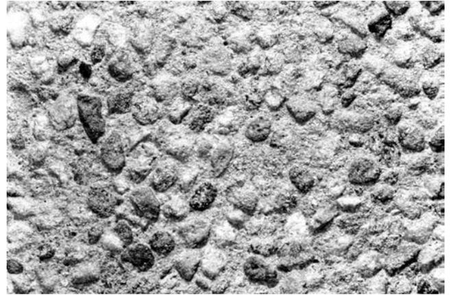
Fig. 6.6.3—Aggregate exposed by sandblasting.
